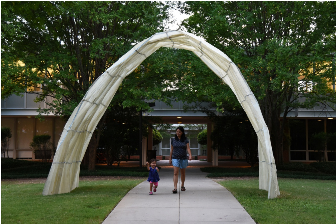
Figure 3: The lightweight folded plate structure spanned 16'.
